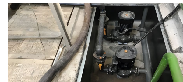
• Reclaimed water delivery pump installed
