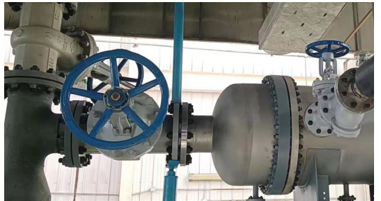
Shell-and-tube Air-to-water Heat Exchanger Added after Renovation
